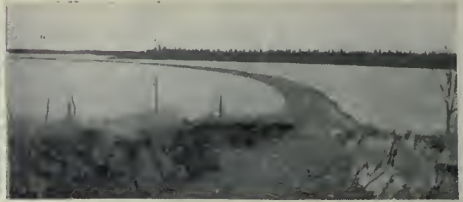
Dyke which diverts Falcon River.
